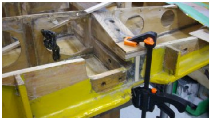
Work in progress on the repair of the wing structure.
